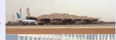
King Khalid International Airport, Riad
