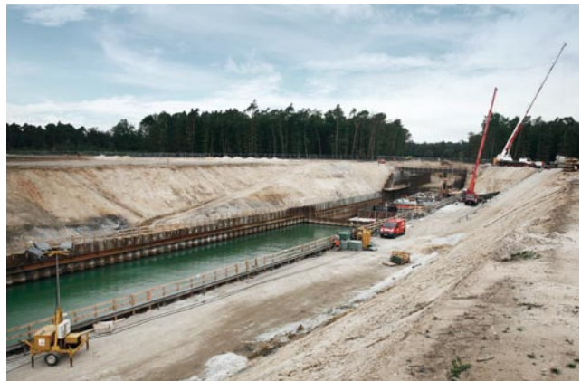
The Okrifteler Street has to be relocated as a tunnel for the new runway.
